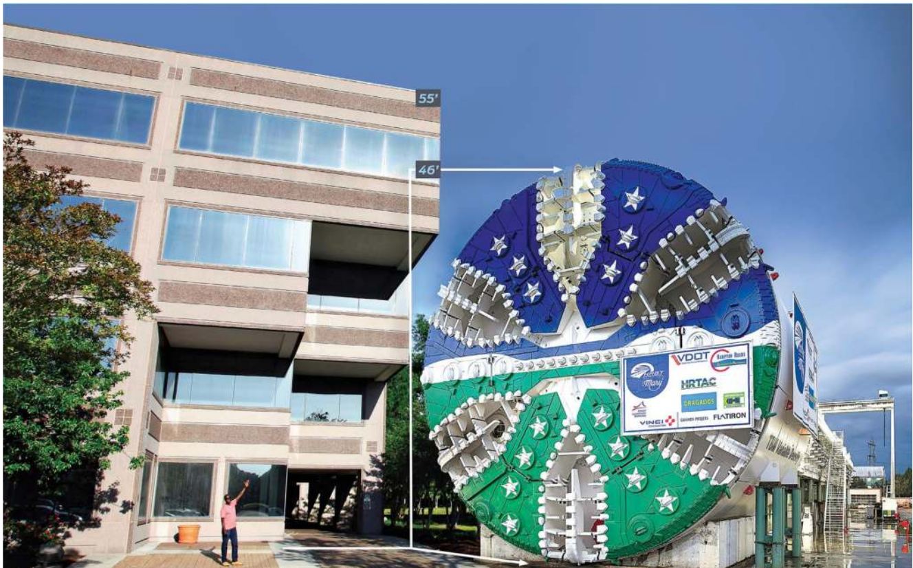
Scale of the TBM next to the HRBT Headquarters
